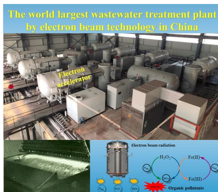
Figure 1. The application of electron beam radiation for the treatment of dyeing wastewater in Jiangmen city, Guangdong province, China
